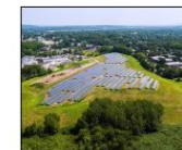
Renewable Energy: Solar array at Rumford Avenue
