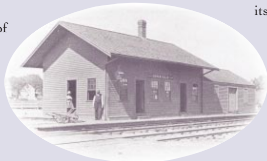
Upper Falls Depot
