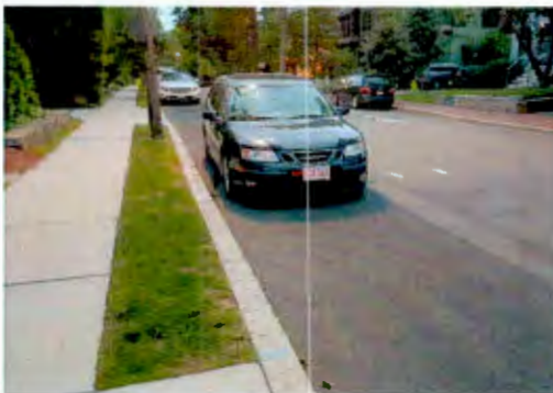
Porous Asphalt Parking Lane Lakeview Ave, Cambridge
