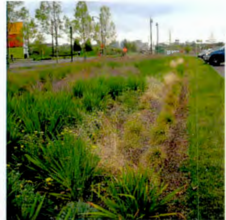
Bioretention Basin Assembly Row, Somerville
