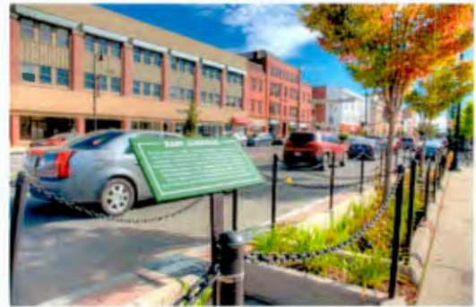
Bioretention Planters North Street, Pittsfield
