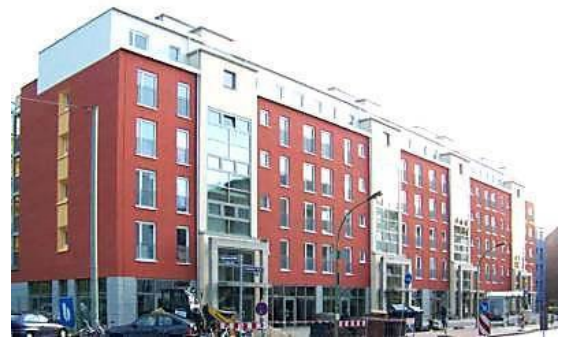
Sophienhof, a multi-family development in Frankfurt, Germany designed to Passive House standards
