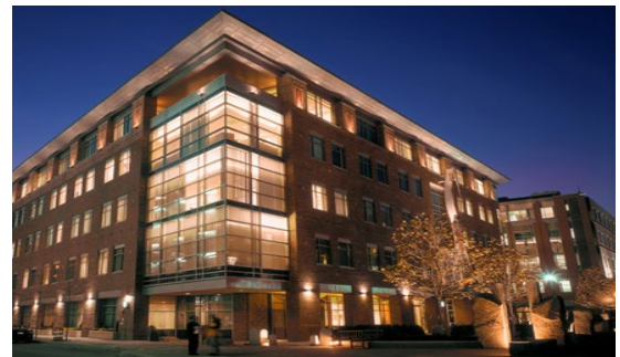
Highlighting architectural features of a building
