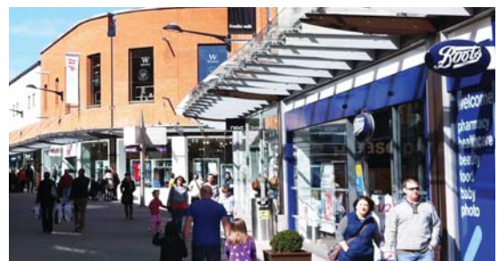
Protective canopies at storefront transition zone
