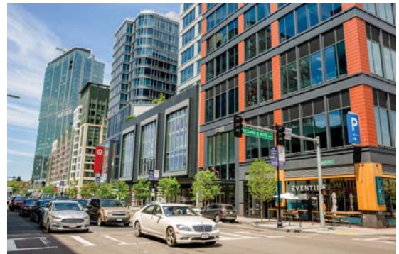
High quality and well-detailed use of materials
