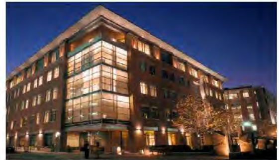
Highlighting architectural features of a building
