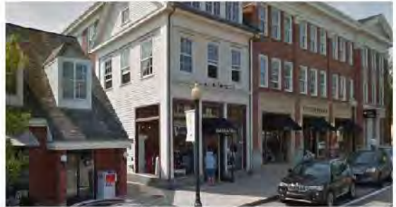
Multiple commercial entries and wrapping storefronts
