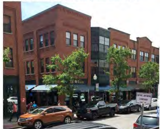
Mixed-use building with well-defined street edge
