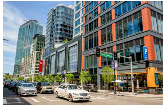
High quality and well-detailed use of materials
