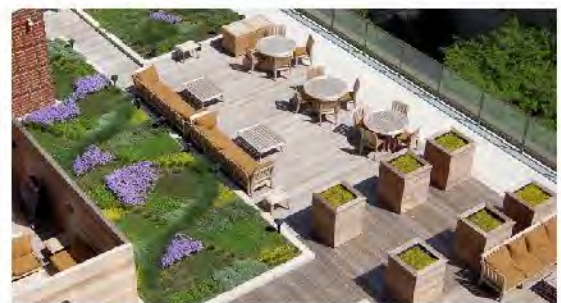
Cluster roof equipment to allow for usable space
