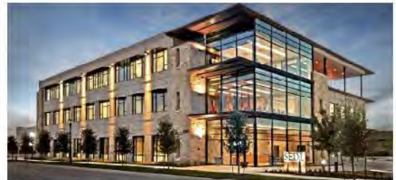
Highlighting architectural features of a building
