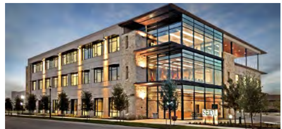
Highlighting architectural features of a building
