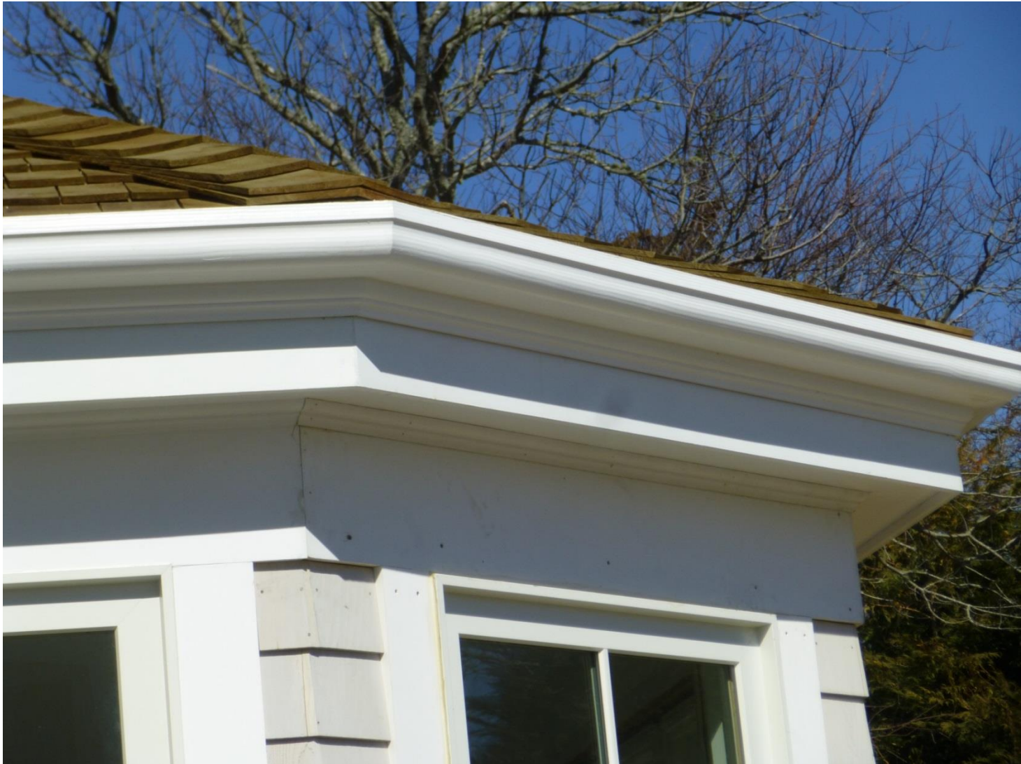
Old Harbor Lane - Chatham, MA
