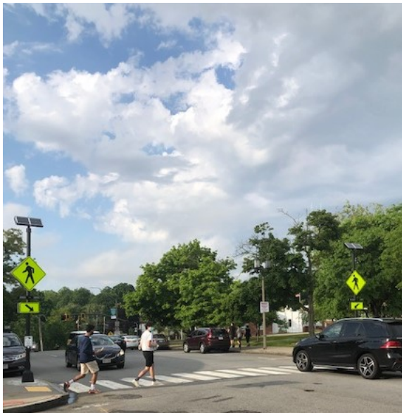
Rectangular Rapid Flashing Beacon at Newton Centre
