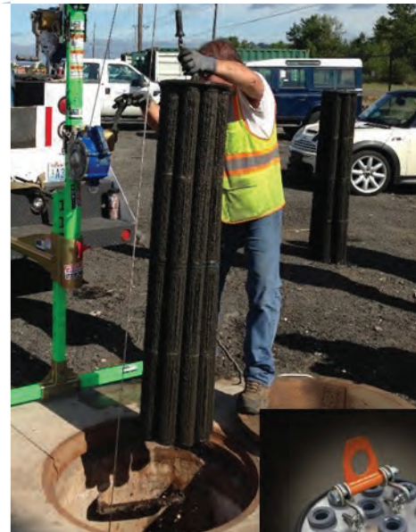
Cartridge Removal & Lifting Device
