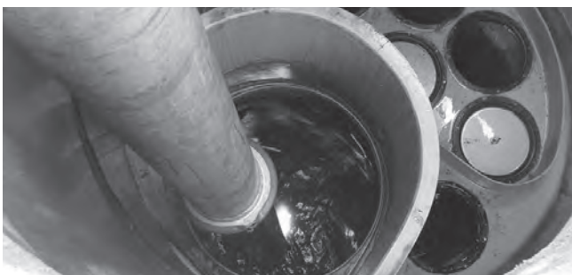
Vacuuming Sump Through MAW
