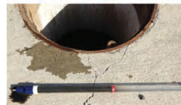
Inspection Utilizing Sediment Probe
