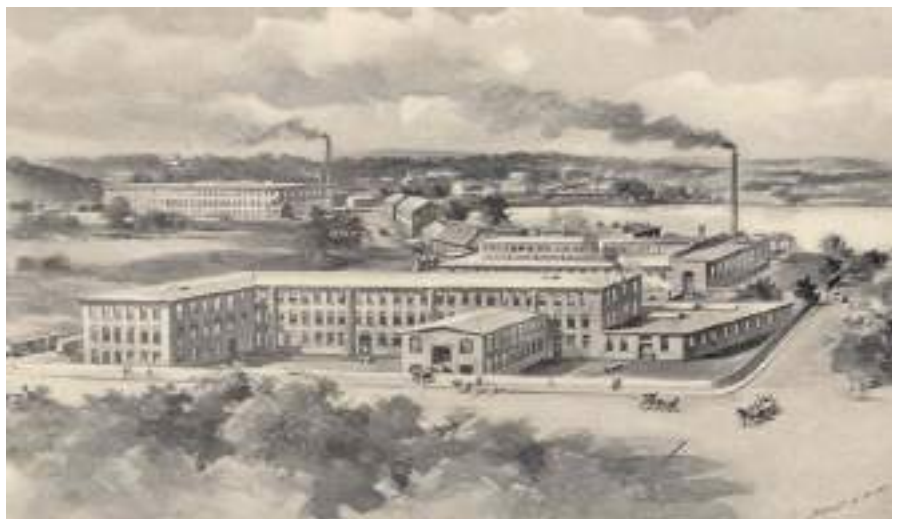
Mill Buildings in Upper Falls (1895)
