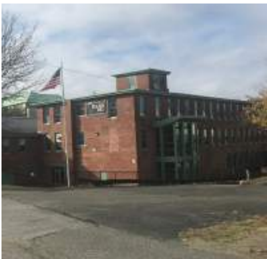
A converted mill building on Needham Street
