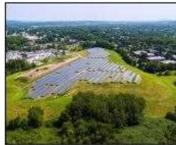
Renewable Energy: Solar array at Rumford Avenue
