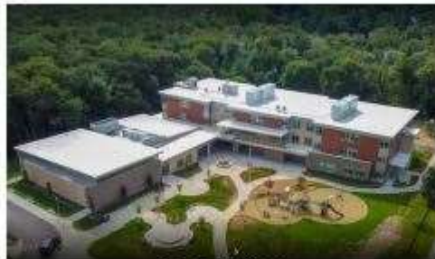
Green Buildings: Zervas Elementary School
