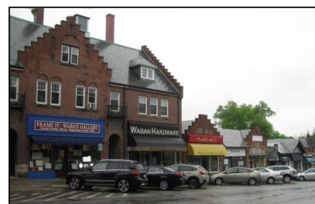
2-12 Windsor Road (1641 Beacon Street)
