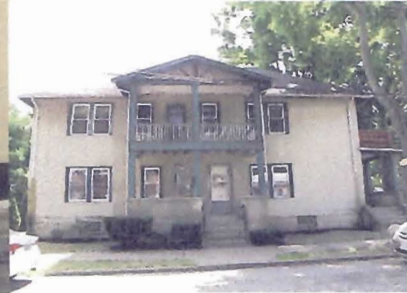
West/Right Side Elevation New windows at left, shorten upper porch, new egress stair from DU-2
