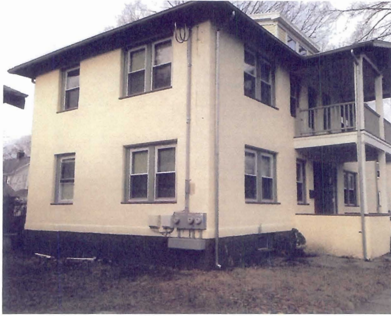
East/Left Side Elevation Masonry restoration.
