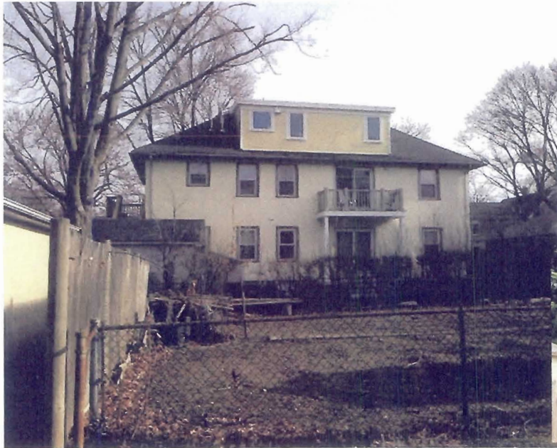
South/Rear Elevation Dormer added, enlarged windows, installed sliding doors, egress porch at DU-1 with open deck at DU-2
