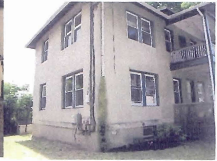
South/Rear Elevation Dormer added, enlarged windows, installed sliding doors, egress porch at DU-1 with open deck at DU-2
