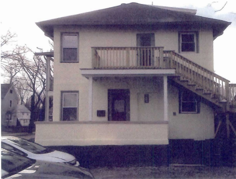
West/Right Side Elevation New windows at left, shorten upper porch, new egress stair from DU-2
