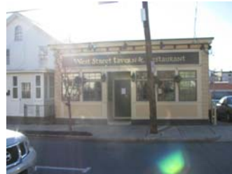
Street Façade of the Building
