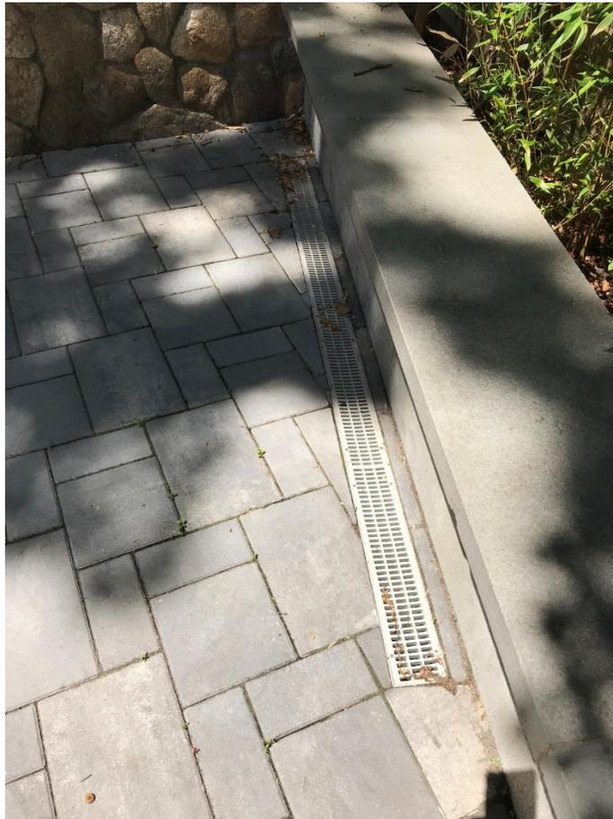
*This area drain was not accounted for in the original drainage calculations*
