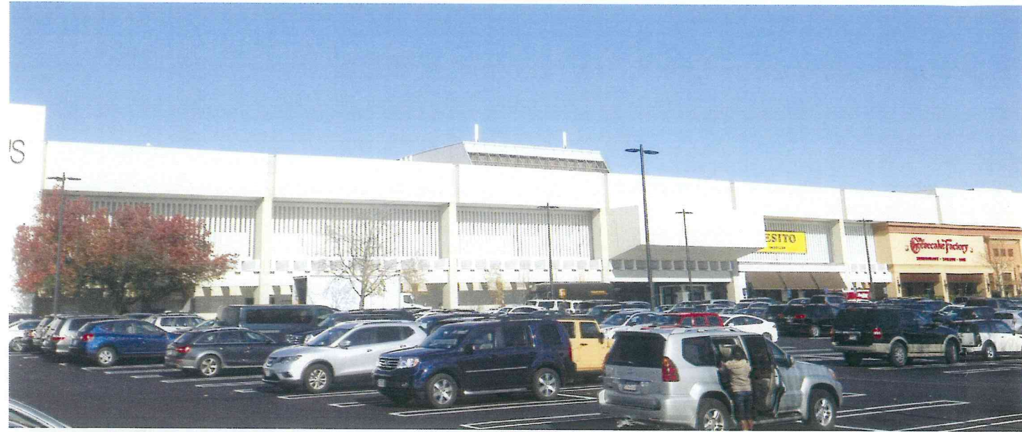
1 MALL FACADE - EXISTING CONDITIONS SCALE: N/A
