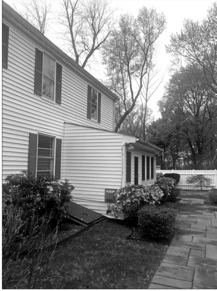
2 EXISTING EXTERIOR VIEW @ NORTH / EAST FACADE 893 WATERTOWN STREET, NEWTON, MA
