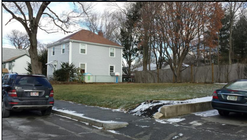
Photo of current conditions
