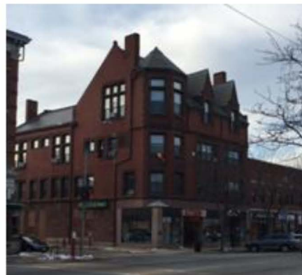
Corner of Summer and Main streets Building
