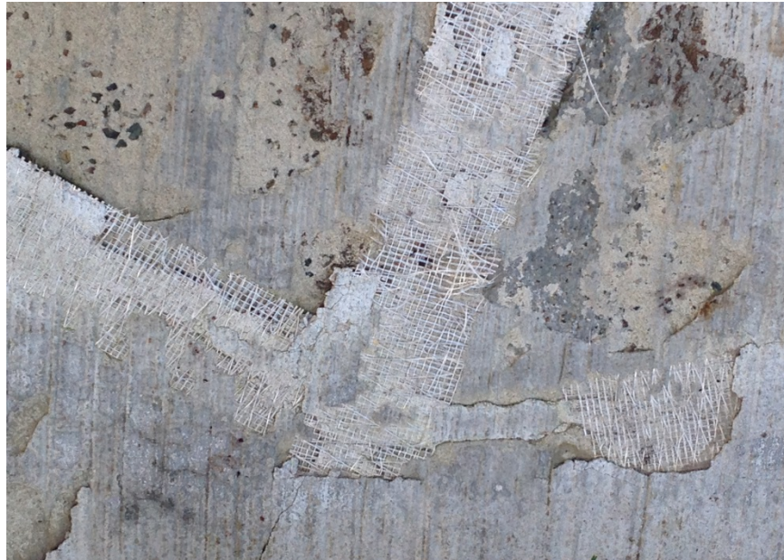
Substandard repair
