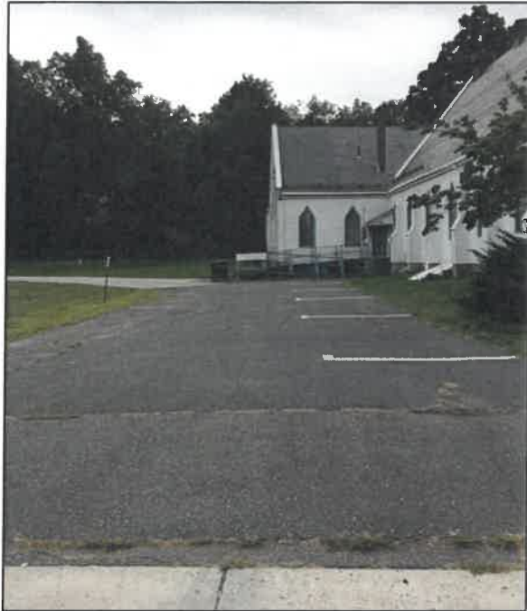
Site Driveway Entrance (from Washington Street) Also Depicting Drop-Off and Pick-Up Parking Spaces
