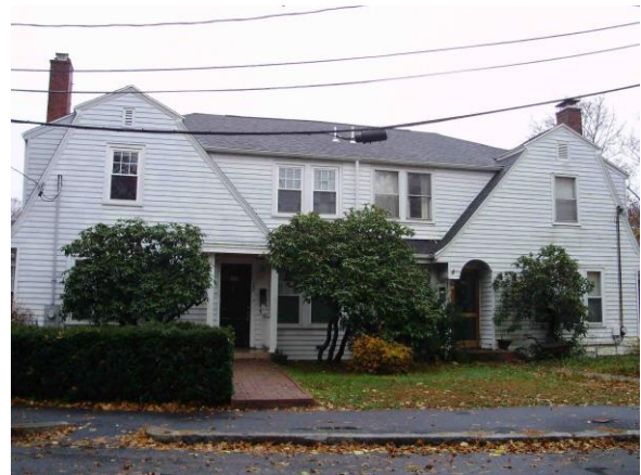
360 Ward Street (left side)
