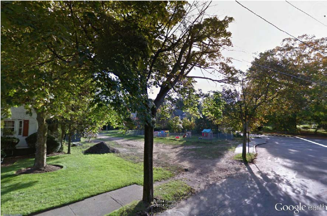
Looking Westerly Missing sidewalk & driveway apron
