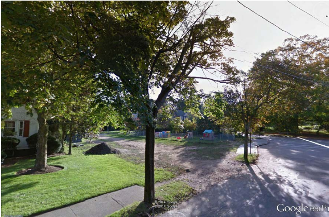
Looking Westerly Missing sidewalk & driveway apron
