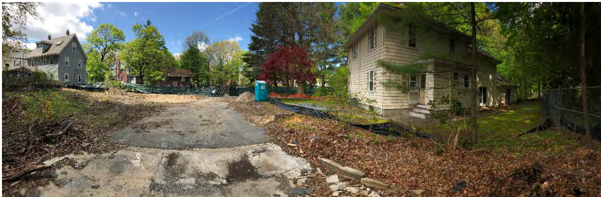
Viewing west towards Walnut Street
