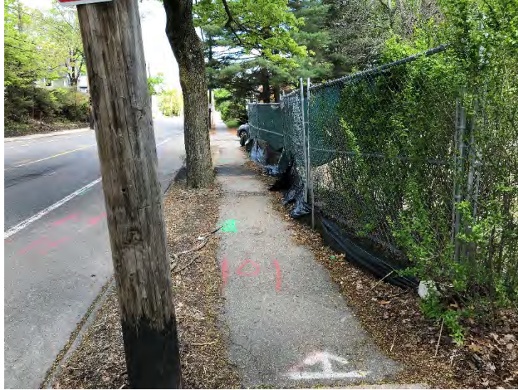
Existing Sidewalk with underground utilities delineated
