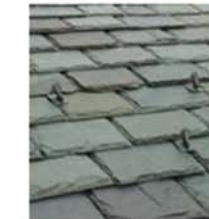
Gutters, Roof, Stone
