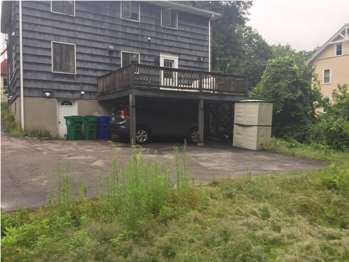
Rear elevation of existing 2 family unit
