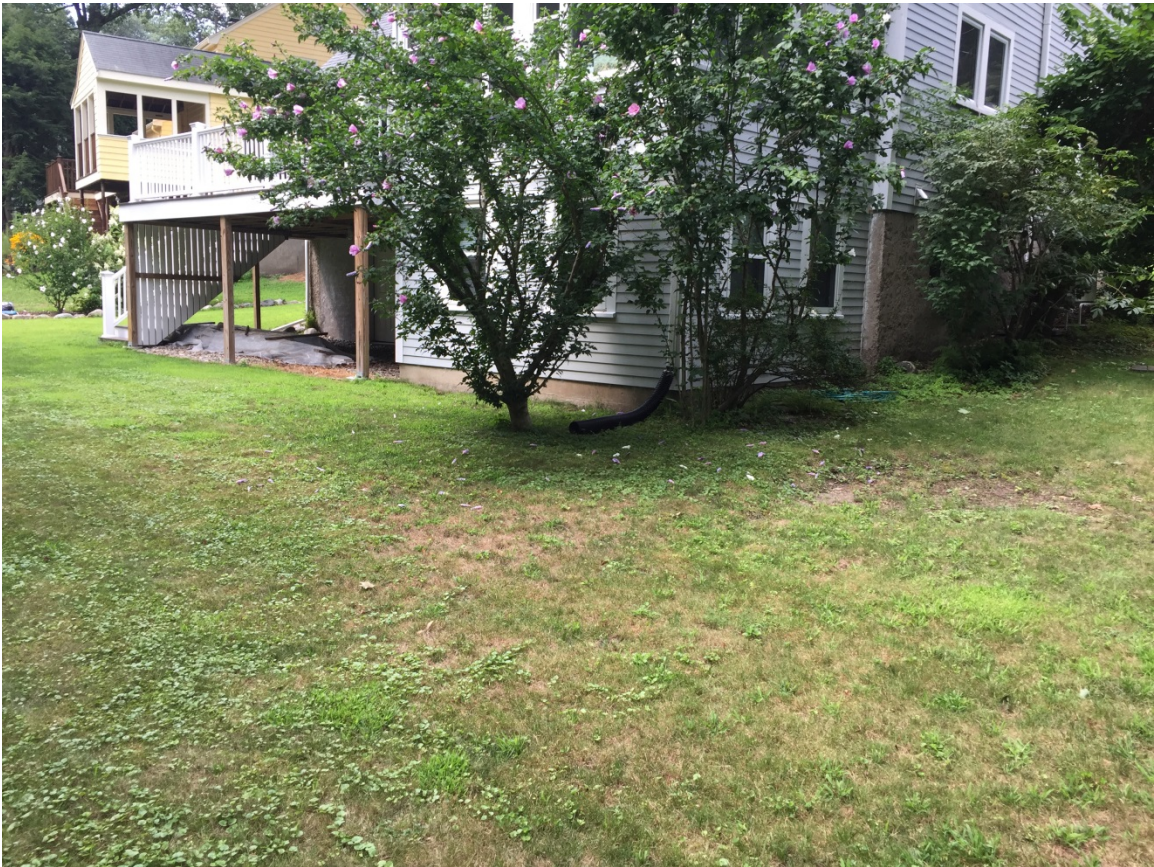
View from the southeastern corner
