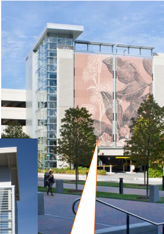
Fabric panels on metal substructure at Cambridge Discovery Park parking garage
