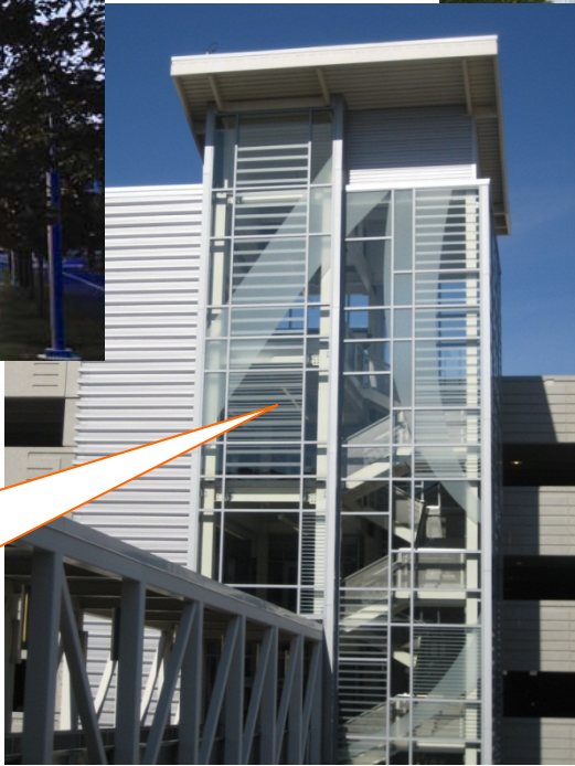
Glass, corrugated metal and patterned precast concrete at the Natick Mall public parking garage
