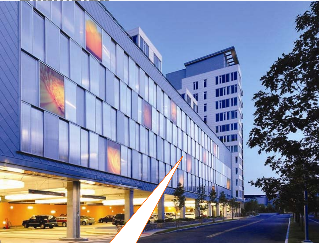
Translucent plastic panels and photographic prints mask the Nouvelle at Natick condominium's garage
