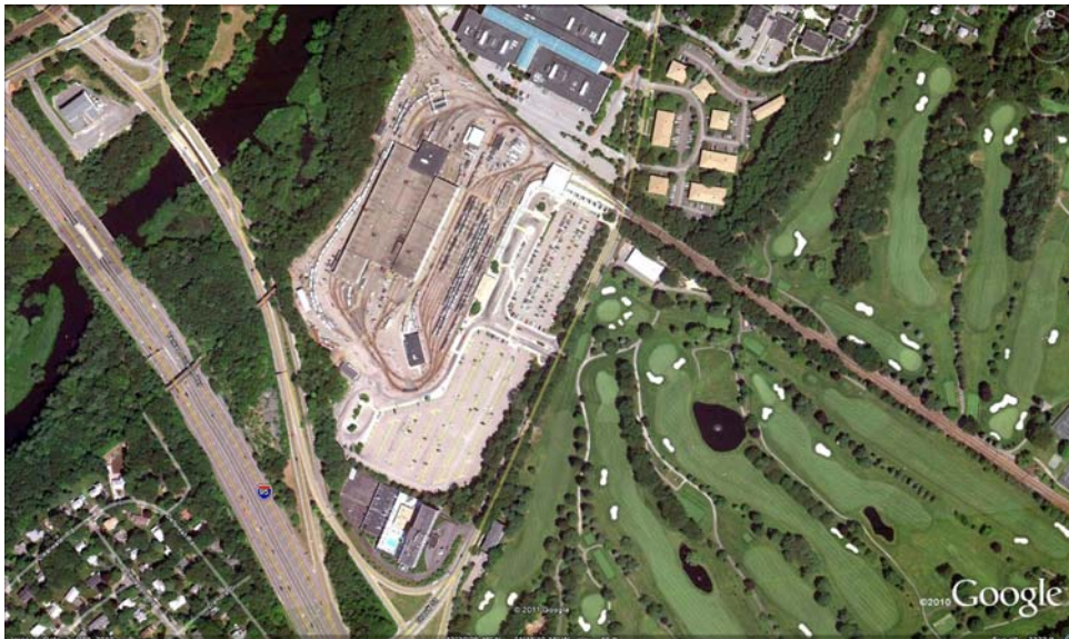
Map 1 – Aerial view of Site of Proposed Riverside Station TOD in Newton, MA
