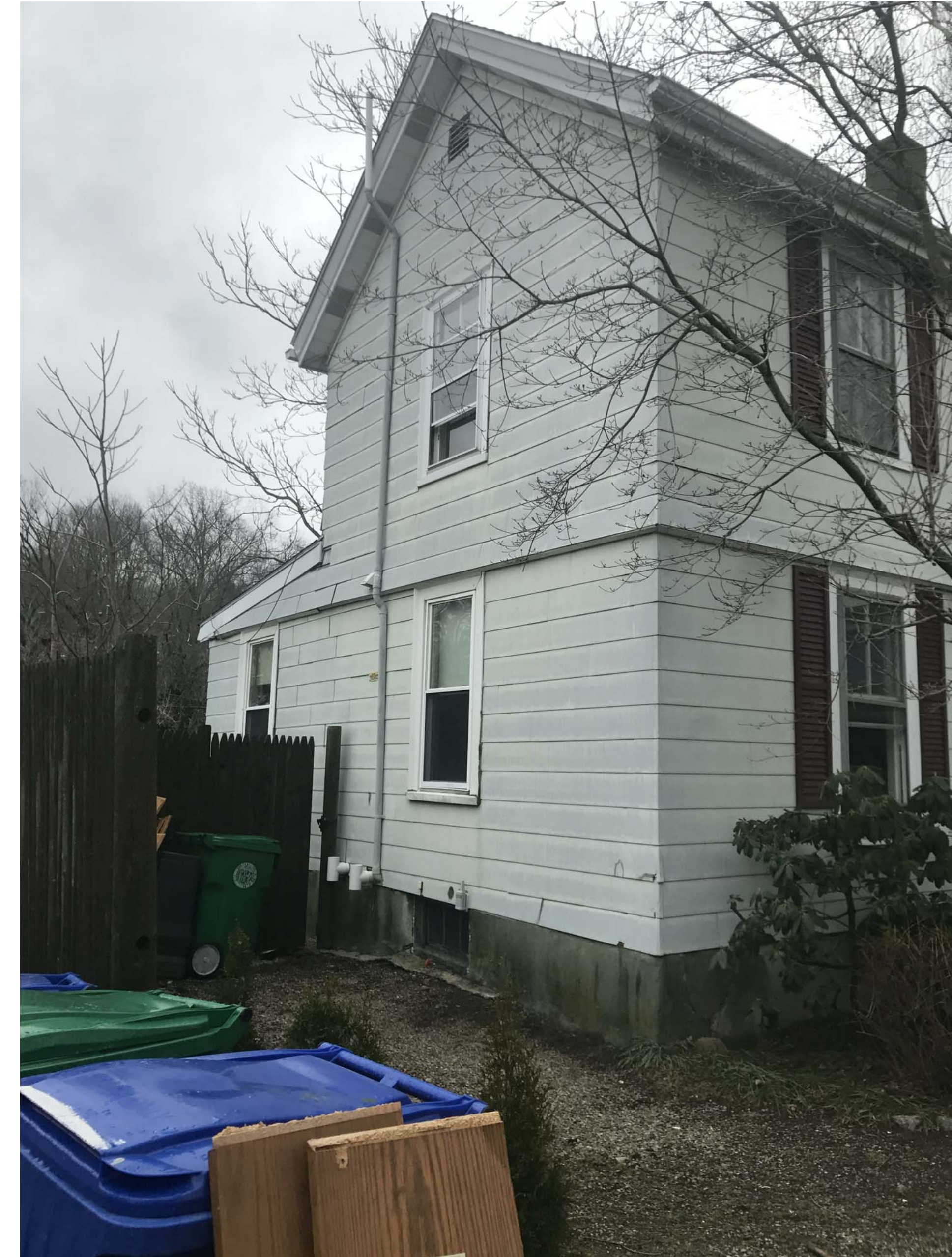
EXISTING BUILDING- LEFT SIDE
