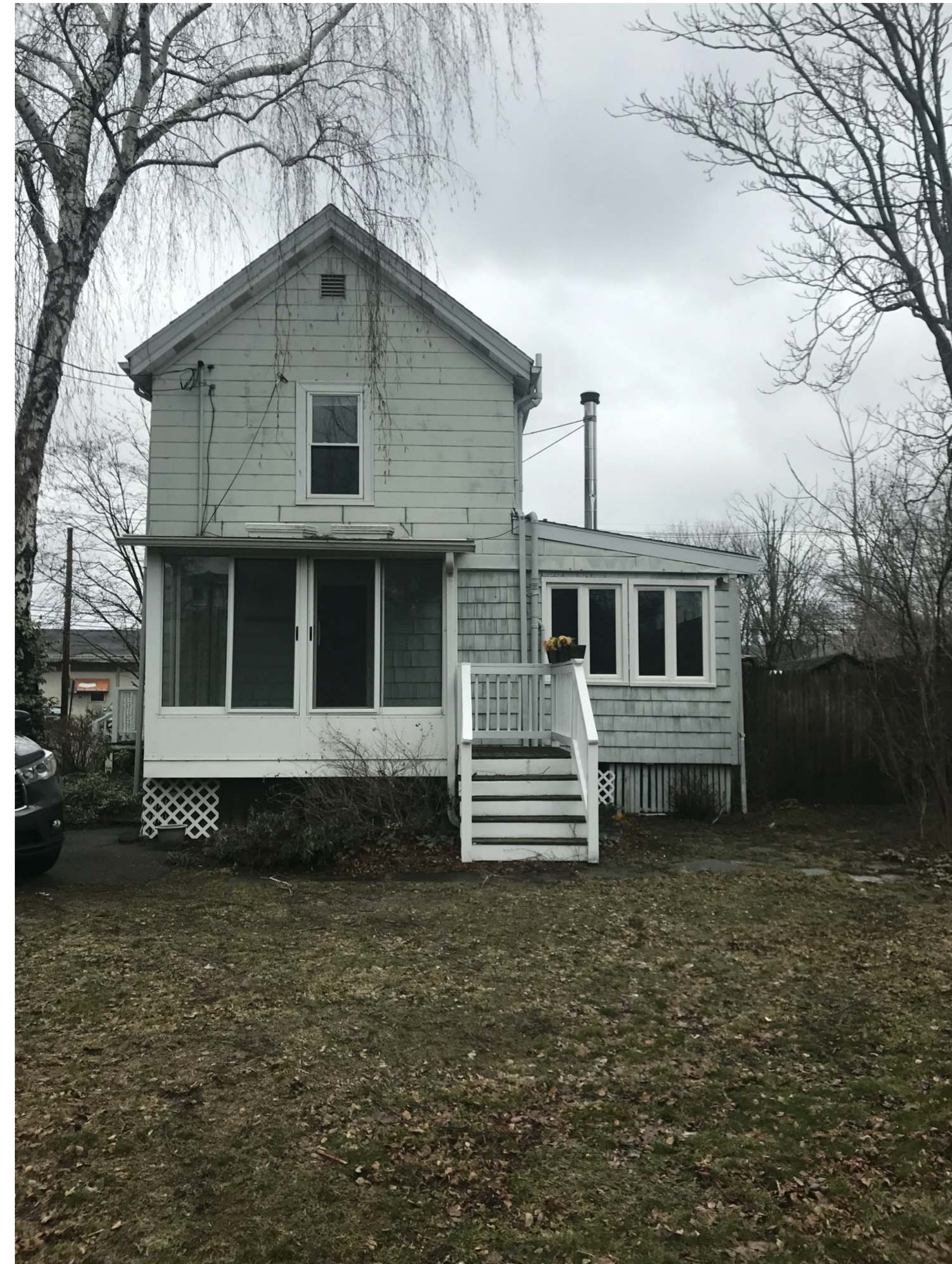
EXISTING BUILDING- RIGHT SIDE
