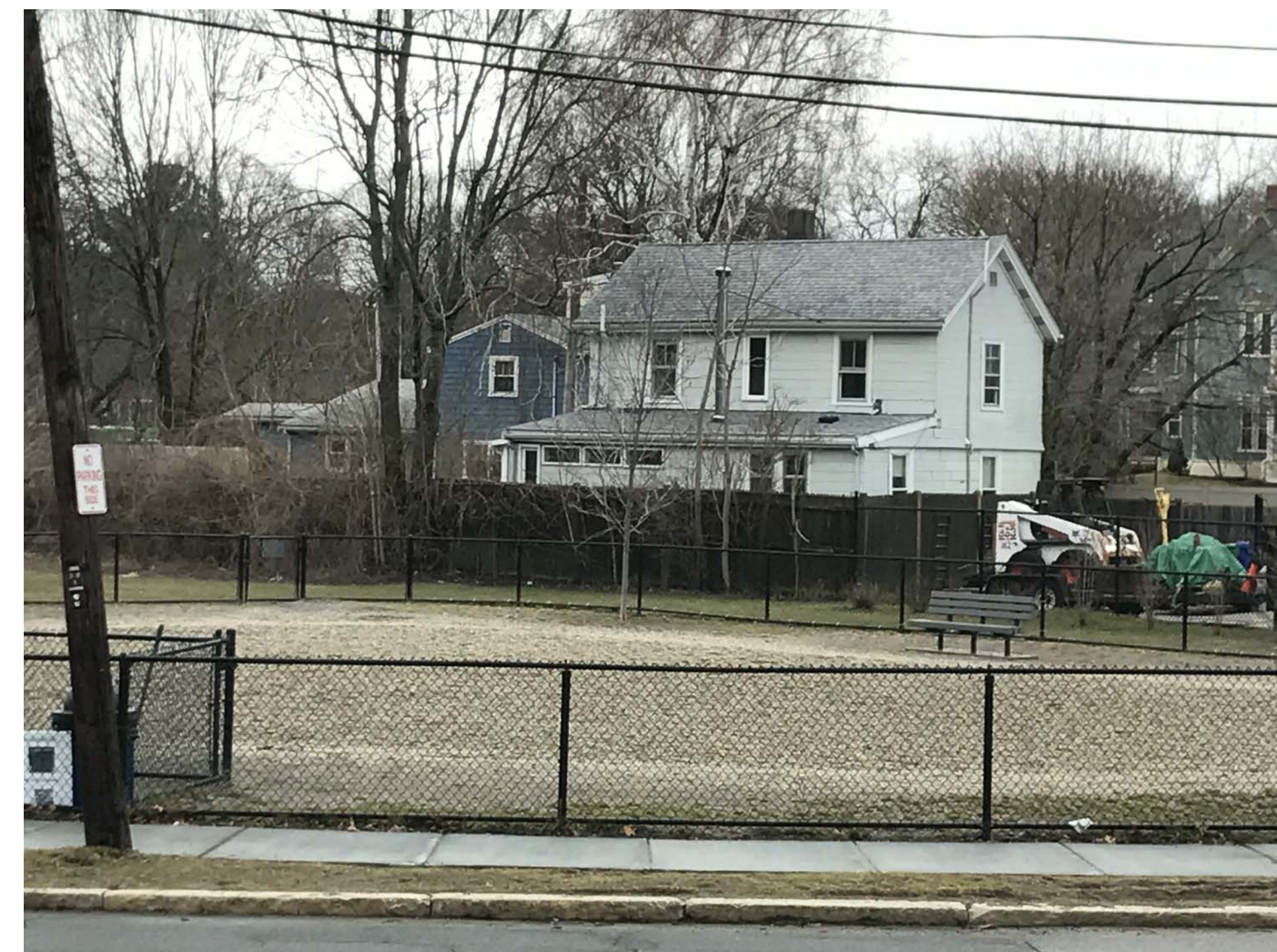
EXISTING BUILDING- REAR
