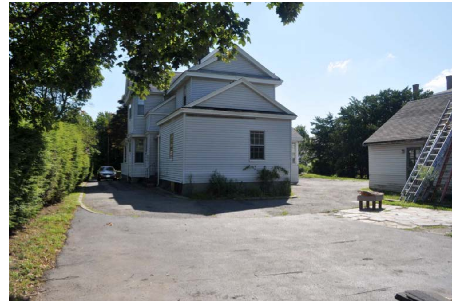
Rear of Existing House
