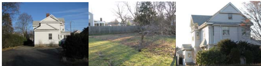
Rear of Existing House
