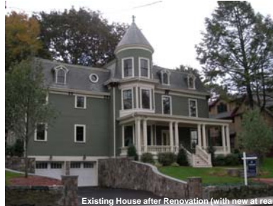
Existing House after Renovation (with new at rear)
