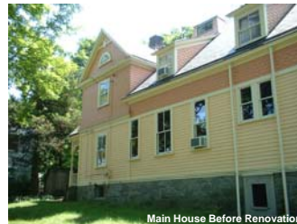
Main House Before Renovation
