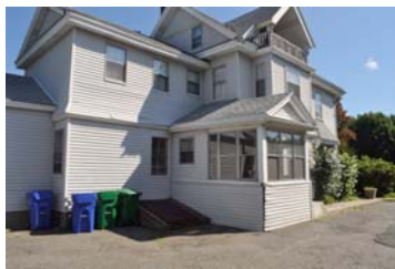
Left Side of Existing House
