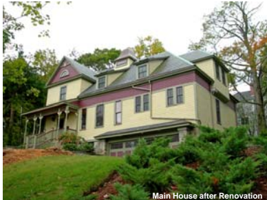
Main House after Renovation
