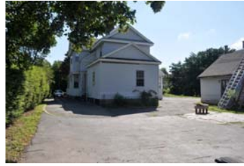
Rear of Existing House
