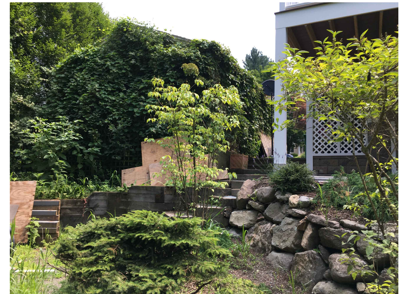
BACK OF GARAGE
