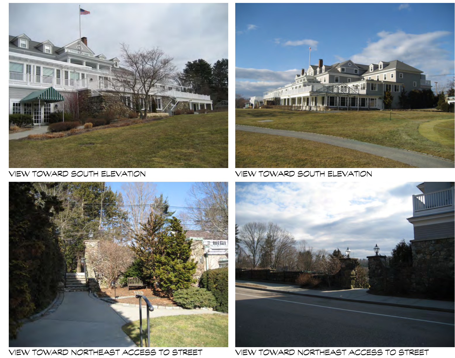
3 EXISTING BUILDING PHOTOS
