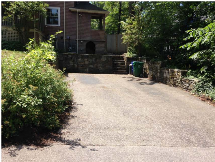
Existing driveway & retaining wall
