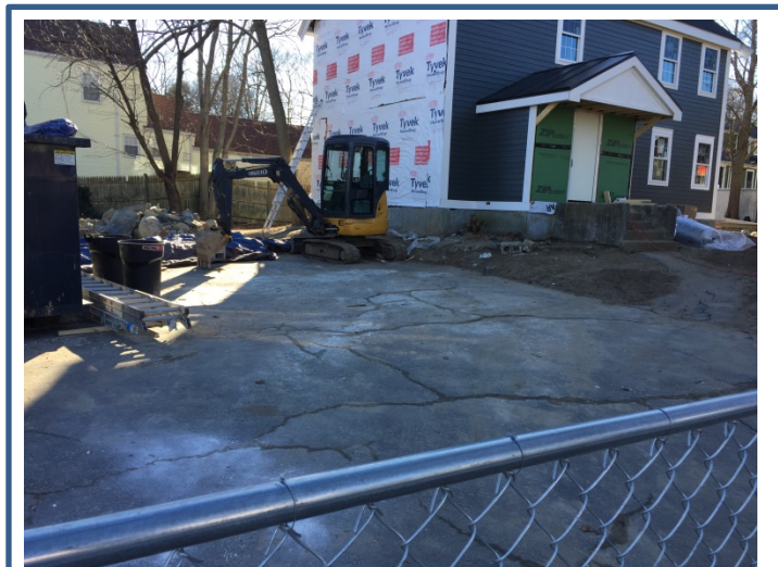
House under renovation
