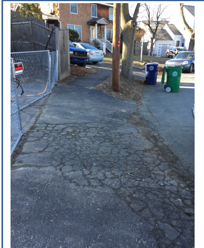
Existing driveway apron
