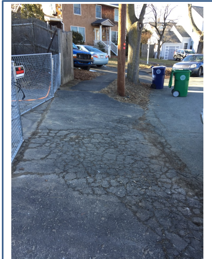
Existing driveway apron
