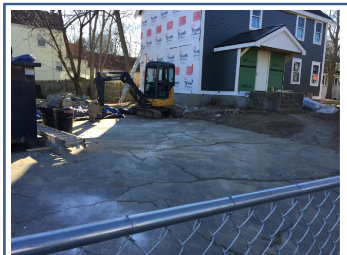
House under renovation
