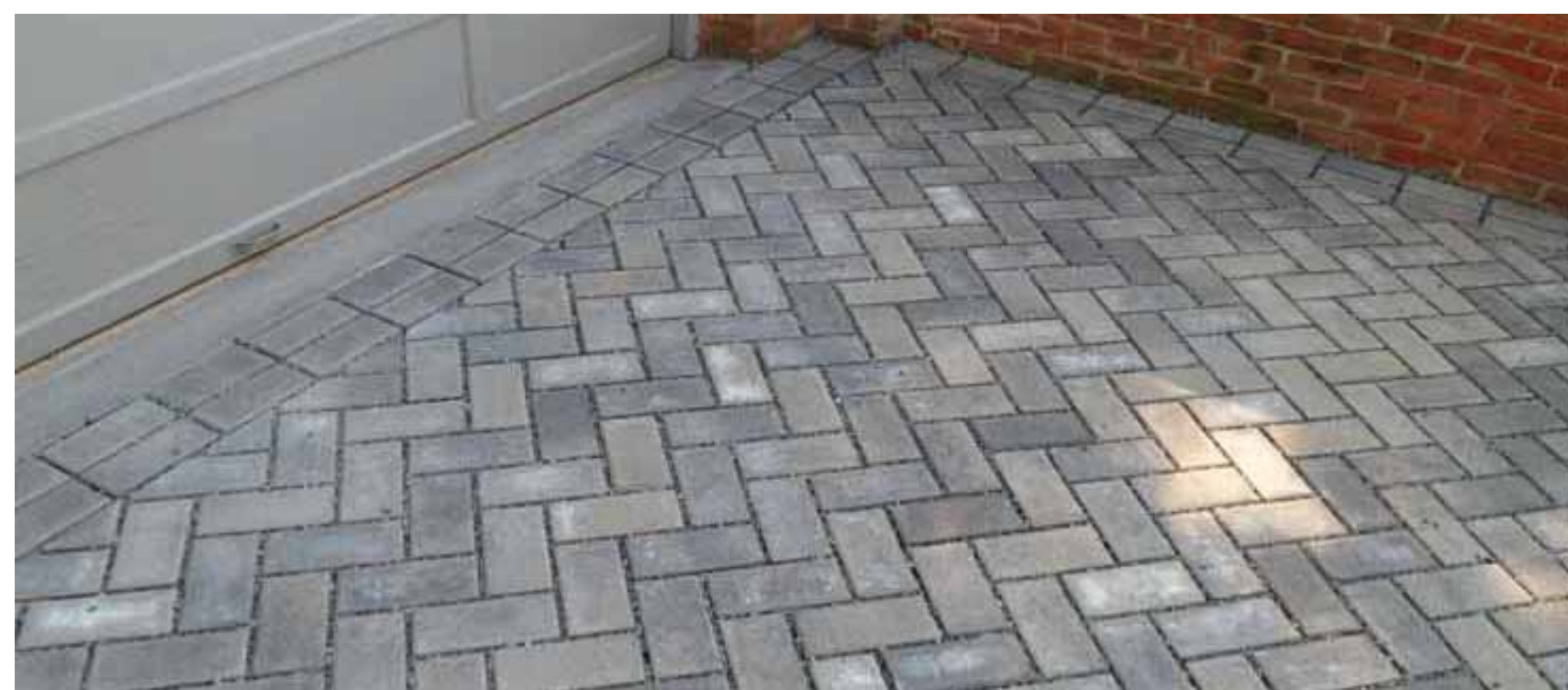
Permeable Driveway Pavers
