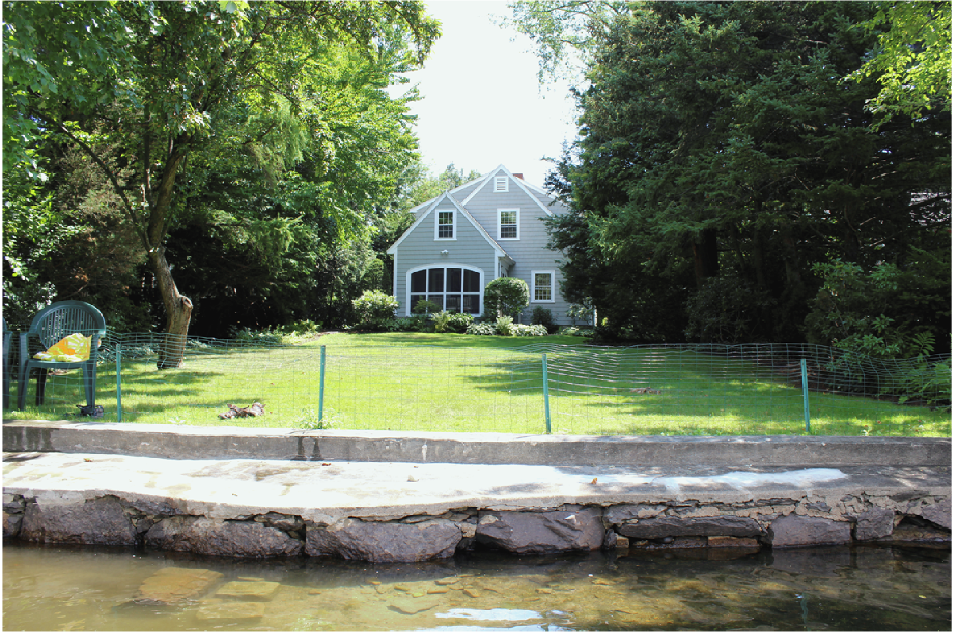
(Photo showing rear of property including the retaining wall along Crystal Lake that is the effective boundary of the property)
