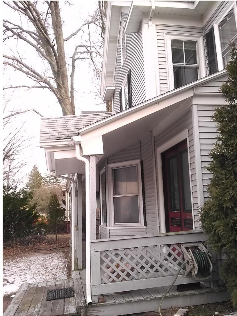
432 NEWTONVILLE AVENUE: ENTRY DETAIL
