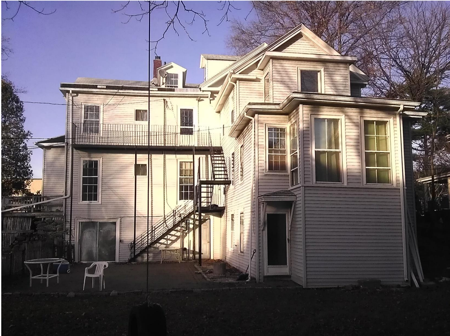
432 NEWTONVILLE AVENUE: SOUTH ELEVATION FROM BACK YARD
