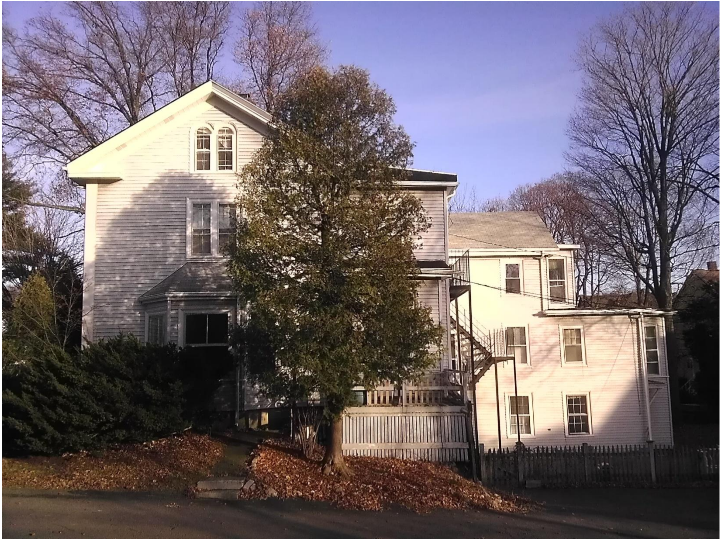
432 NEWTONVILLE AVENUE: WEST ELEVATION FROM PARKING
