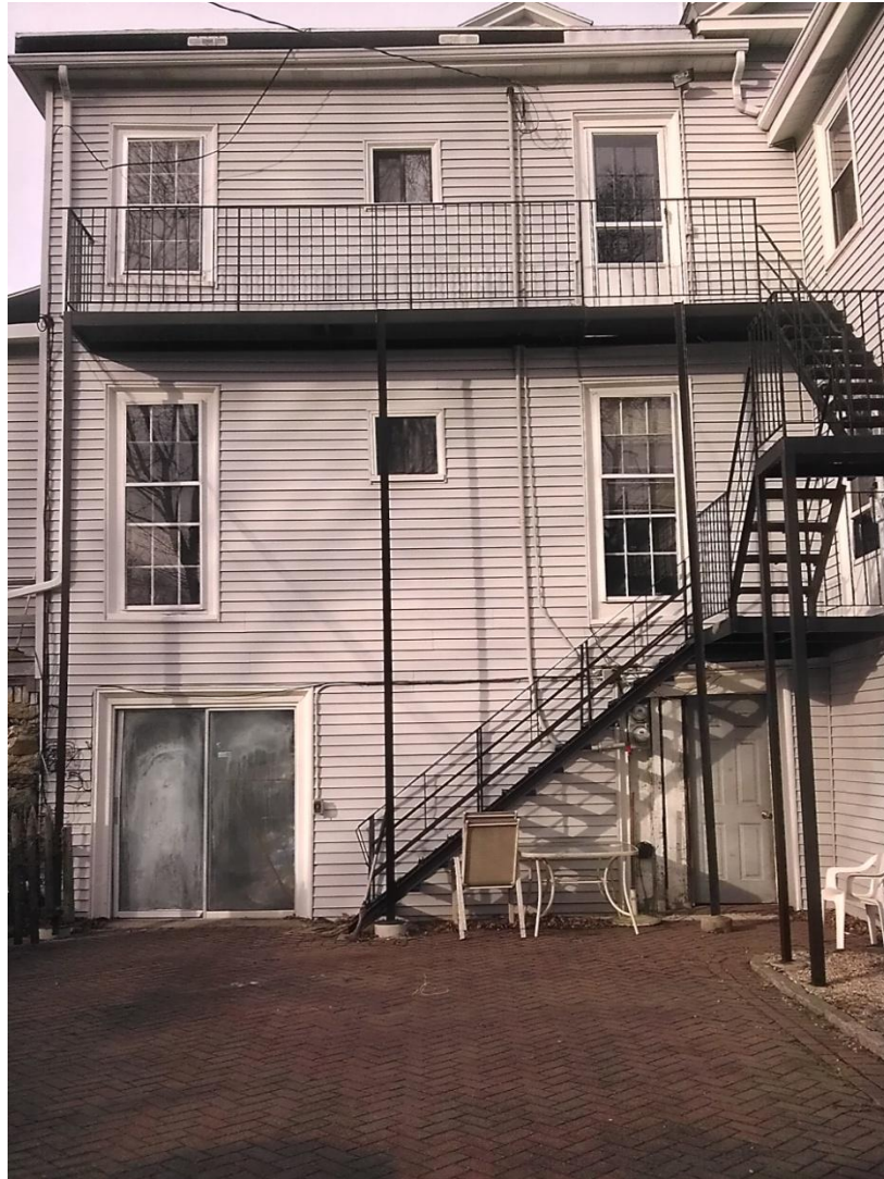
432 NEWTONVILLE AVENUE: INNER CORNER DETAIL
