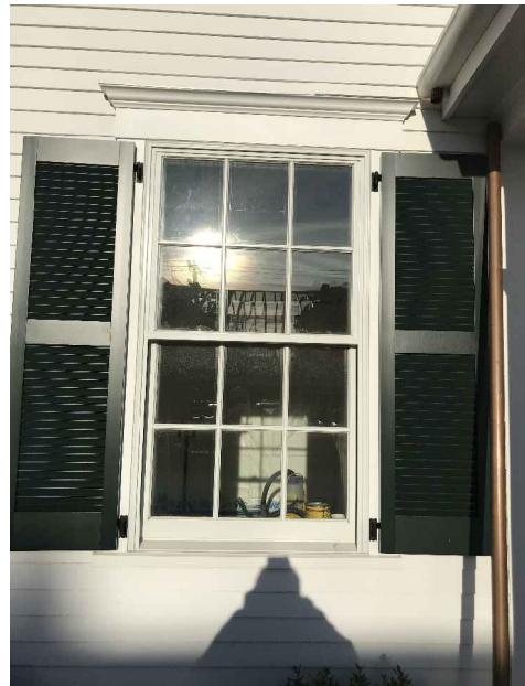
3 ARCHITECT SERIES DOUBLE HUNG WINDOWS NO SCALE
