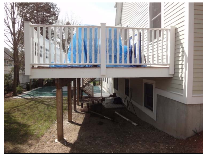
SIDE VIEW OF DECK LOOKING WEST
