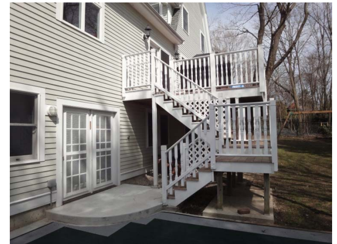
SIDE VIEW OF DECK – LOOKING EAST
