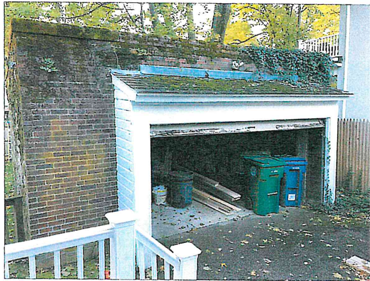
4 GARAGE - FRONT CORNER
