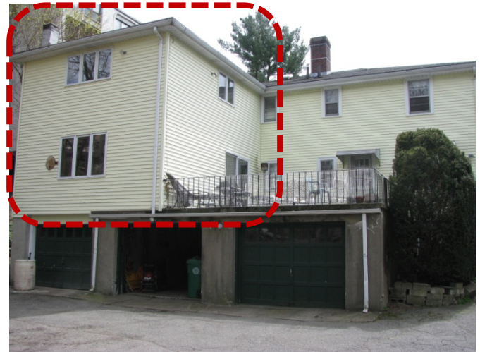
Location of the Proposed Unit (rear of building)
