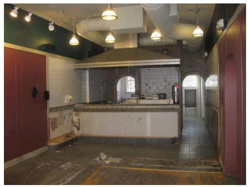
EXISTING CONDITIONS - PHOTO I
