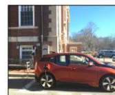
Clean vehicles: City Hall EV charging station
