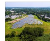
Renewable Energy: Solar array at Rumford Avenue
