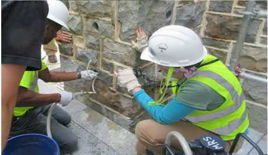
Stabilization – secure exterior stone back to core structure with specialty stone anchorage system
