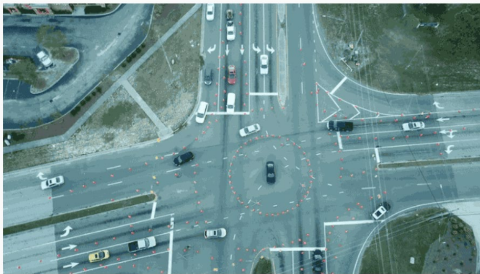
Figure 14. Temporary Roundabout Construction Wilmington NC
